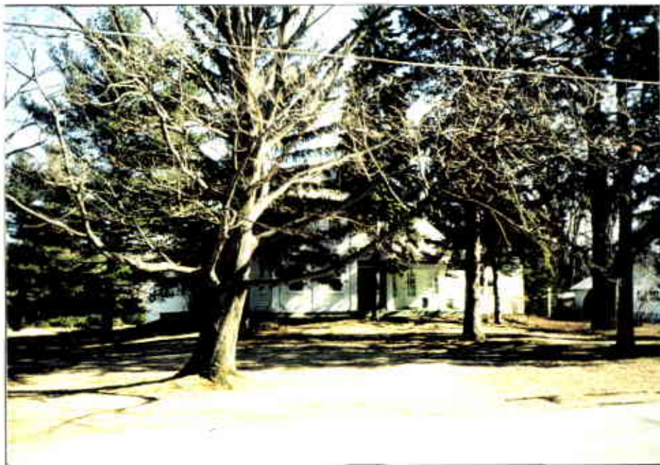
Photo 5 -View of the John V.A. Lansing Farmhouse from Consaul Road.
