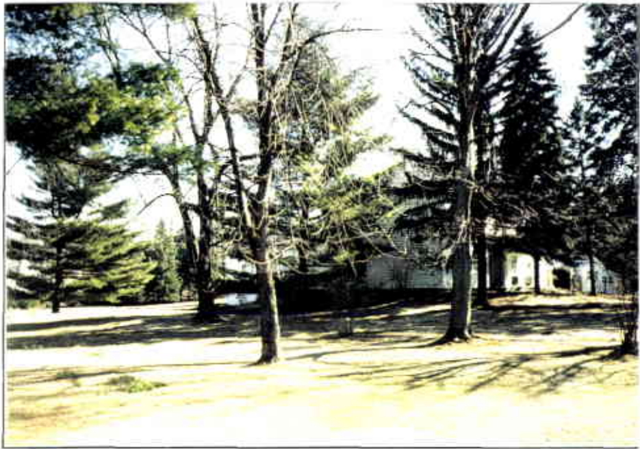
Photo 6 - View of the John V.A. Lansing Farmhouse from Consaul Road.
